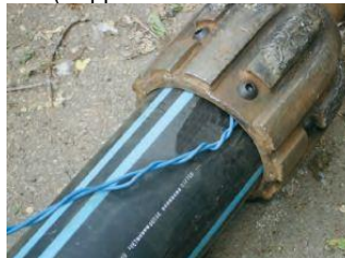
Figure 2 – “Blue” Tracer Wire
