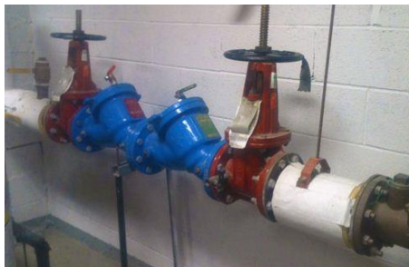
Figure 3 – Example of a Backflow Prevention Assembly
